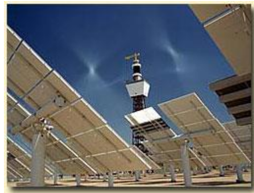
Fig.5 Power tower system
