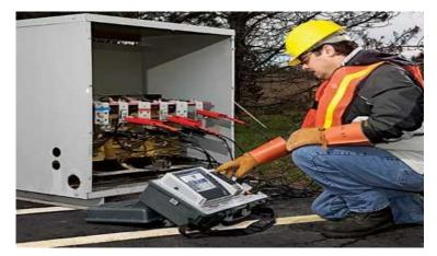
Fig.1. Linemen trying to measure the various parameters of the transformer.
