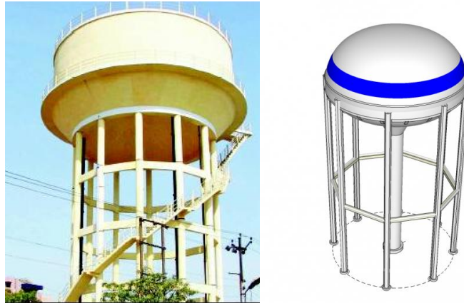
Figure (d): Intze type Water tank Figure (e): Spherical type water tank
