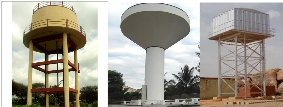
Figure (a): Circular type tank Figure (b): Conical Type water tank Figure (c) : Rectangular type
