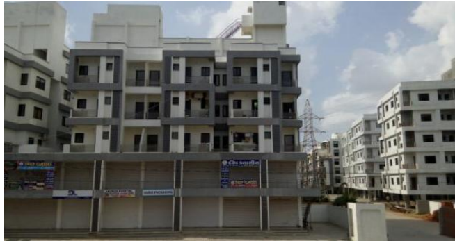
. Fig. 1 layout & Photographic view of Low-rise Building
