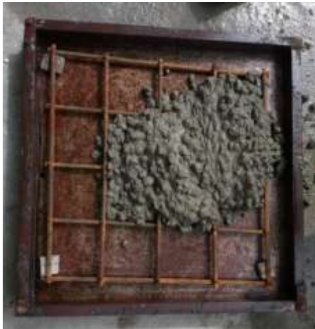
plate 6: Slab mould with reinforcement
