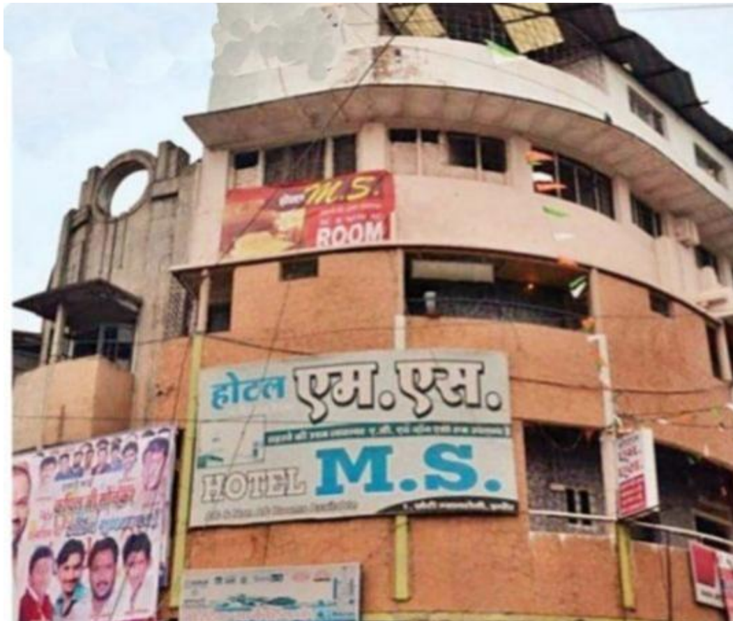
Fig. 6 General view of M.S. Hotel before the collapse
