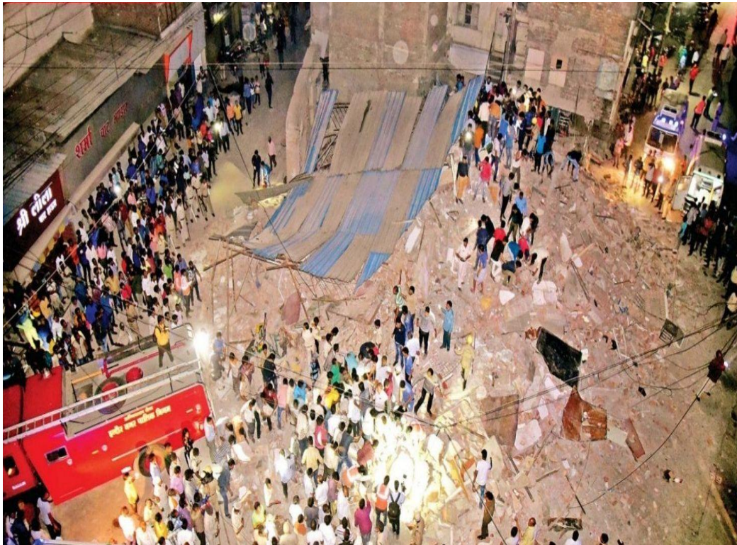
Fig. 7 M.S. Hotel after the collapse
