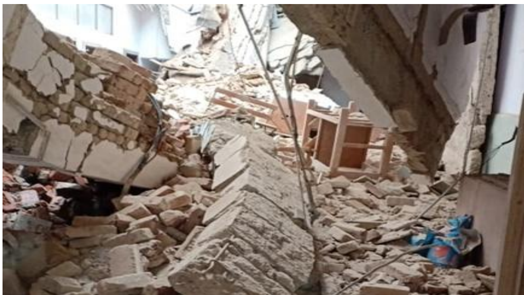
Fig. 11 Condition of structure
