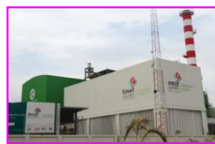
Incineration Plant, Jabalpur
