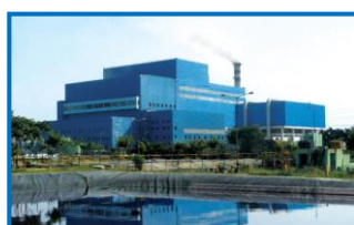
RDF Plant, Narela
