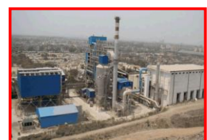
RDF Plant, Ghazipur
