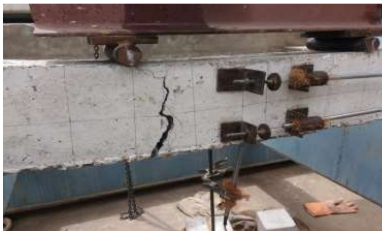
Fig 2 Crack Pattern for the Beam With 100% Lapping
