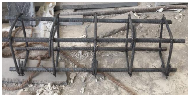
Figure 2: Beam Reinforcement with vertical Stirrups
