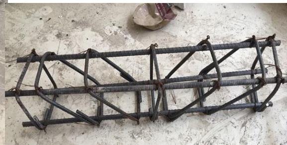
Figure 3: Beam Reinforcement with Inclined Stirrups
