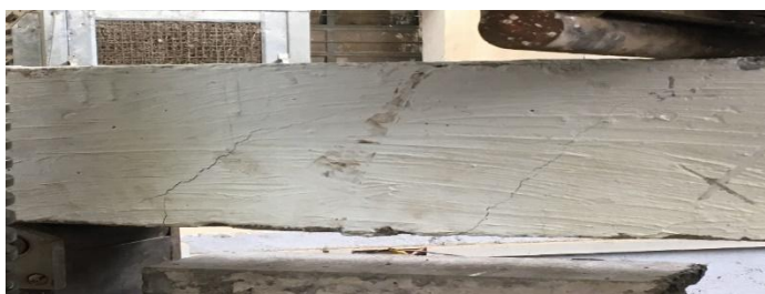
Figure 8: Crack found on RCC beam using inclined stirrups
