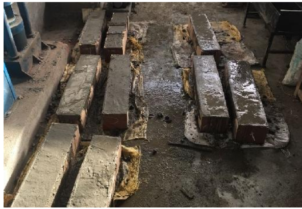
Figure 5: Casting of Reinforced concrete beam
