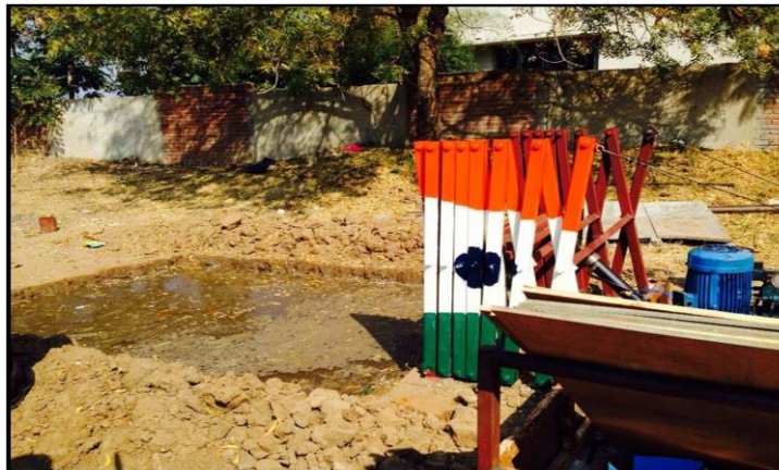
Fig-2-Folding Bridge(Folded Condition)
