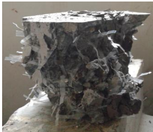
Fig. 3. PET fiber reinforced cube after failure
