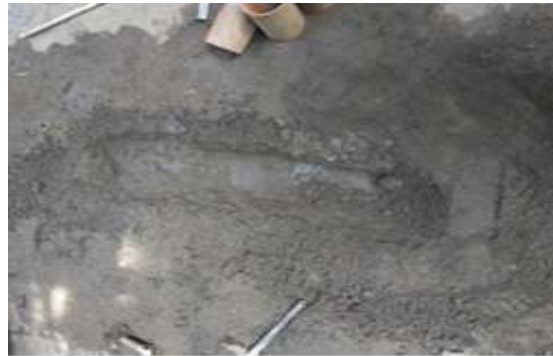
Fig :Preparation of Sand
