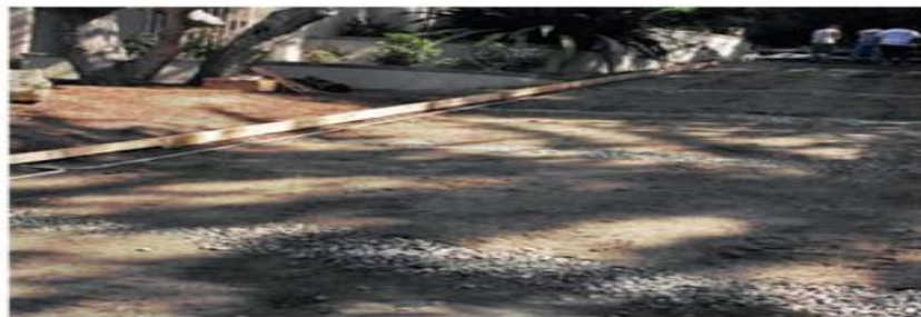
Fig: Sloped Pervious Concrete Pavement with Dug Trenches Filled with Stone
