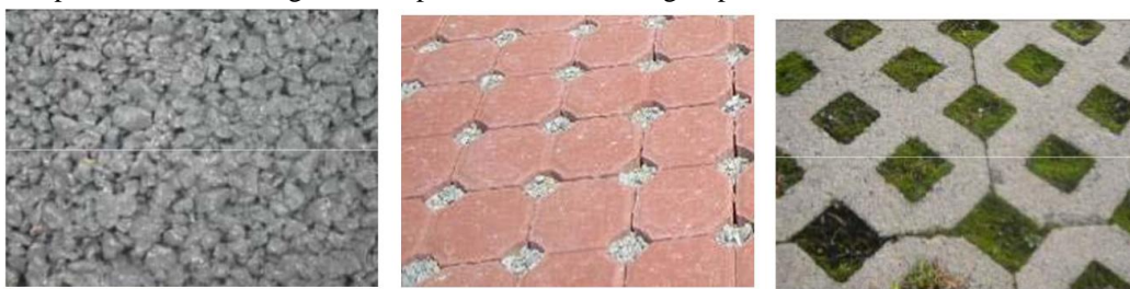
Fig:a. Pervious Concrete, b. Pervious Interlocking Concrete Pavers, c. Concrete Grid Pavers
