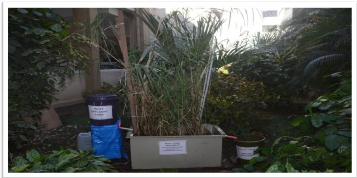
Figure 1: View showing complete constructed/Fabricated Root Zone Treatment technology system.
