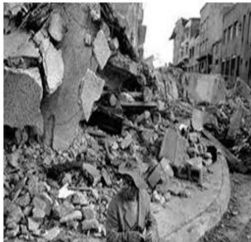
Fig. 7 Total collapse of the building in Rat Islands
