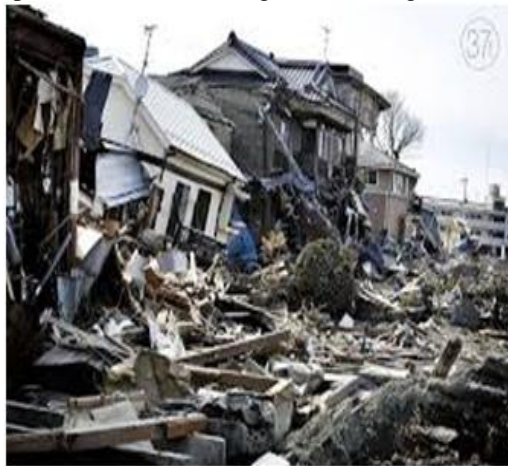
Fig.3 Pounding failure in Tohoku Earthquake
