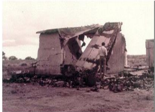
Fig. 10 Collapse of brick masonry structure in Killari Earthquake
