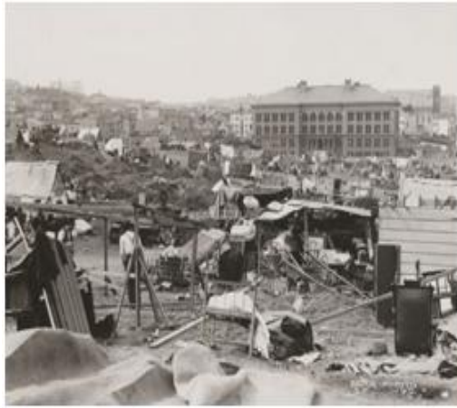
Fig. 6 Partially collapse of the building in Ecuador–Colombia Earthquake.
