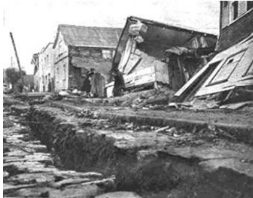
Fig. 1 Partially collapse of the building in Valdivia Earthquake.
