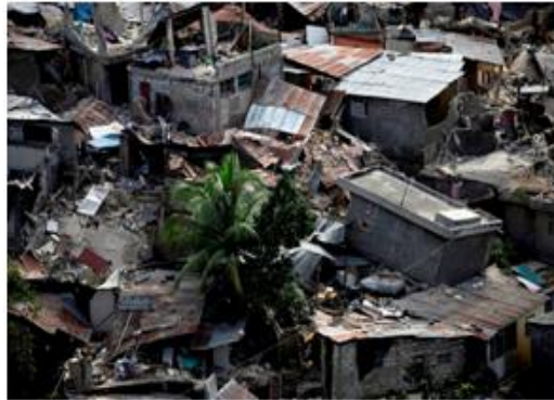
Fig. 8 Partially collapsed of the building in Assam-Tibet Earthquake.
