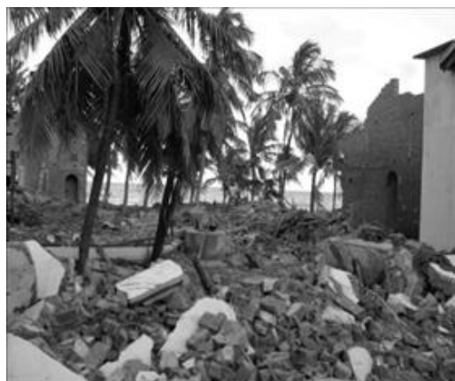
Fig. 2 Total collapse of the building in Sumatra Earthquake
