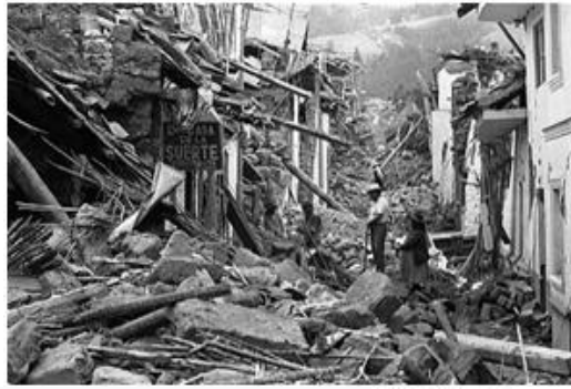
Fig.4 Total collapse of the building in Kamchatka Earthquake.
