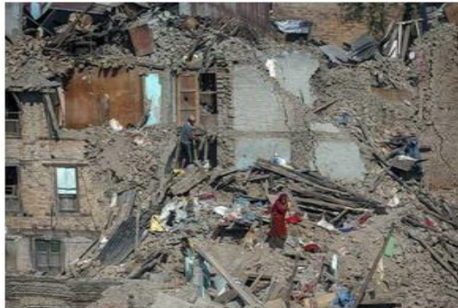
Fig. 21 Quality of mortar and bricks used in building in Nepal Earthquake
