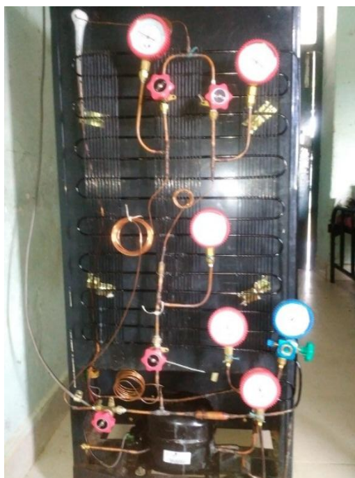
Fig 3 Experimental setup of refrigeration system after using different capillary tube daimeters
