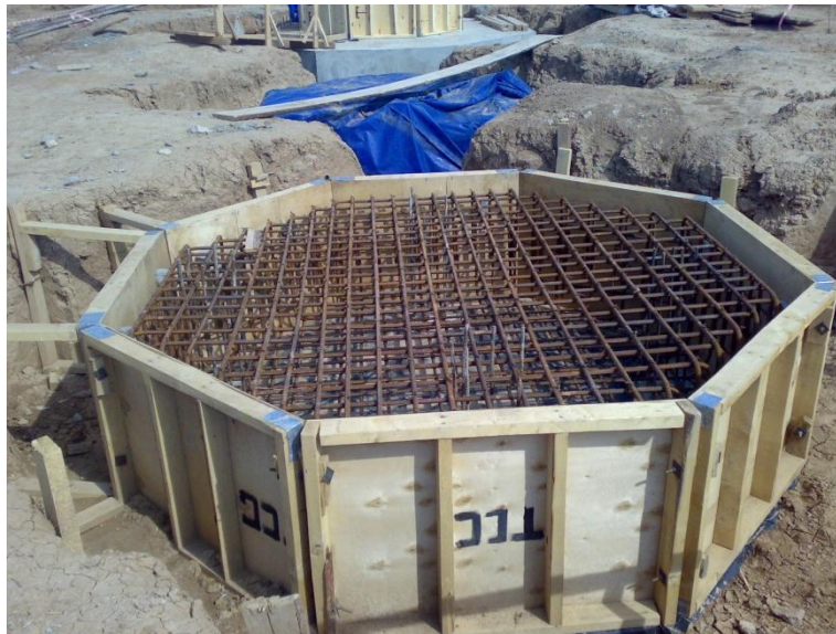
FIG 1.1 Construction of Vertical Vessel Foundation (Octagonal)
