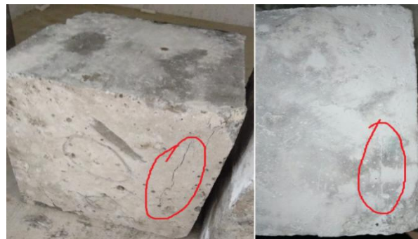
Fig 5 The concrete cube before and after the self healing process
