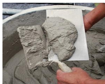
Fig 3. Mixing of Fly ash Aggregate Ingredients in Concrete Mixer
