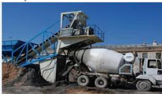
Figure 7: Showing the Volume Batching
