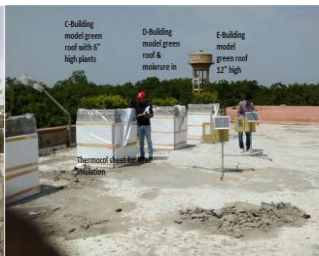
Figure No 9 Block E, D, C test cell ( 1m x 1m x 1m ) green roofs covered with thermocol sheet
