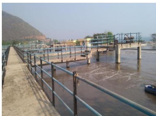
Fig:1 25 MLD Capacity Sewage treatment plant, Visakhapatnam
