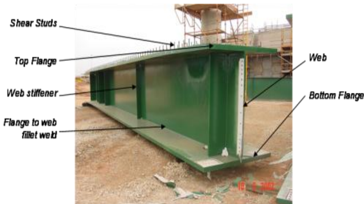
Figure-1 Typical Elevation of a Plate Girder
