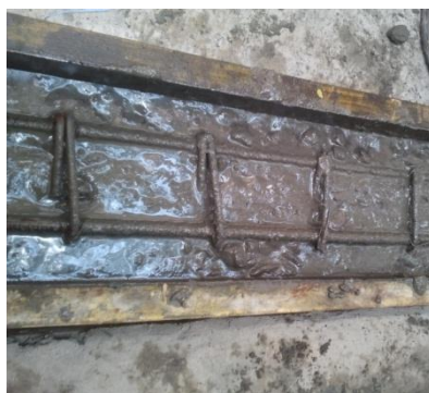
Fig 4 : Casting of Beams
