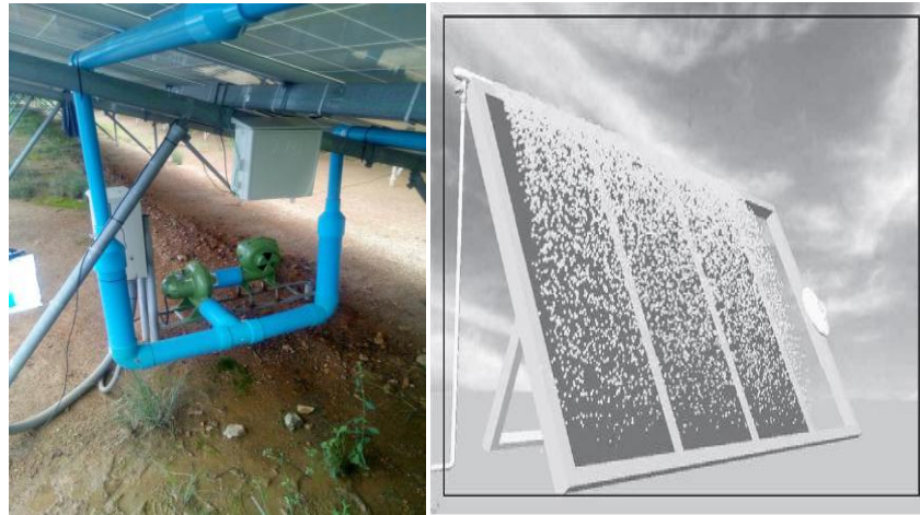
FIG 4 WATER COOLING SYSTEM.
