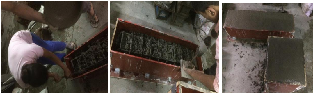
Fig. 1 Casting Of Beams &Columns
